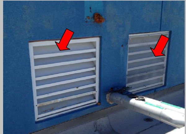
Photo #14 Louvers at mechanical openings.
