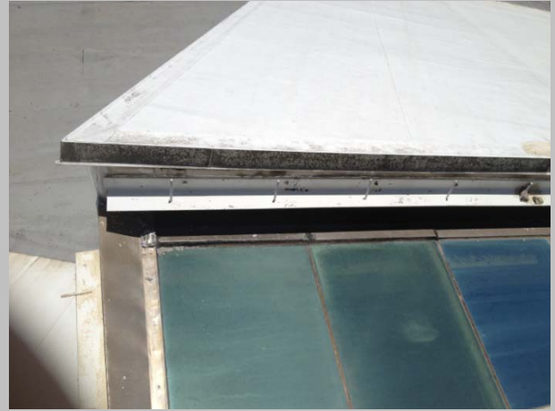
Photo #8 Gutter system at central canopy/main lobby skylight.
