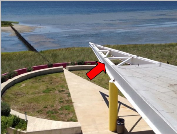
Photo #15 West side central canopy
