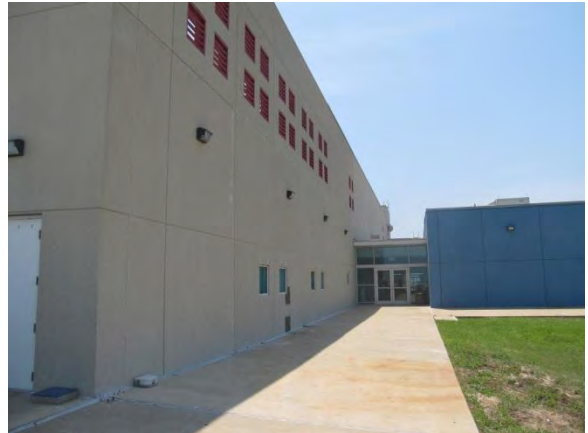
Photo #38 Northwest elevation facing south.
