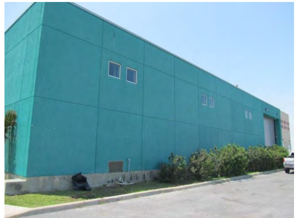
Photo #24 North elevation.
