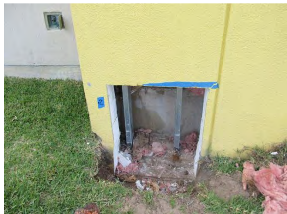
Photo #5 DTO #2 - Taken along east elevation.
