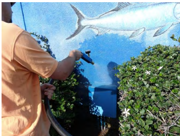
Photo #17 Water spray testing in progress to electrical box.
