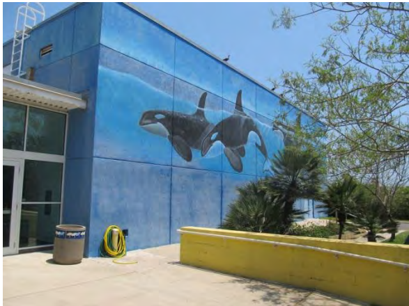
Photo #53 South elevation facing northeast.
