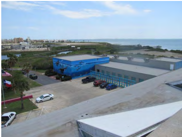
Photo #67 Overview of roof areas facing southwest.
