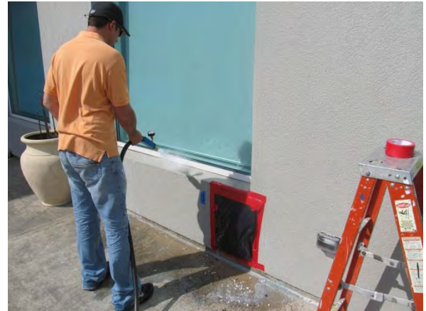
Photo #2 Water spray testing in progress along window sill.
