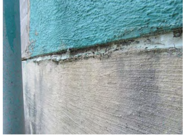
Photo #26 Joint between EIFS and foundation.
