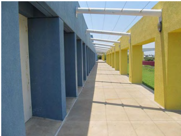
Photo #47 Overview of west elevation facing south.
