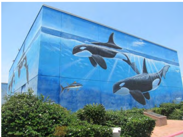
Photo #59 East "WyLand" wall.
