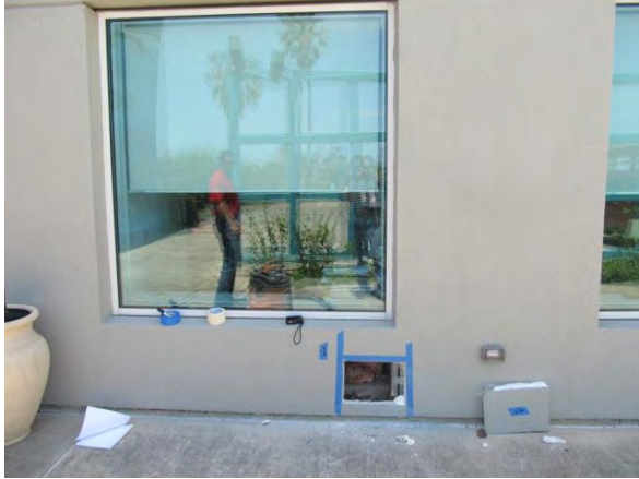
Photo #1 DTO #1 – Taken along east elevation.
