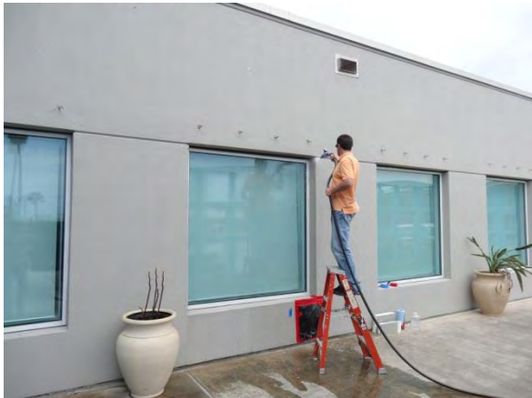
Photo #3 Water spray testing in progress along window head/jamb.
