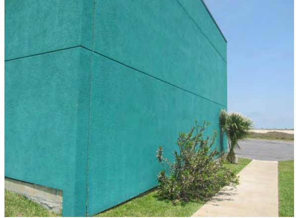
Photo #20 East elevation of Green Room facing north.
