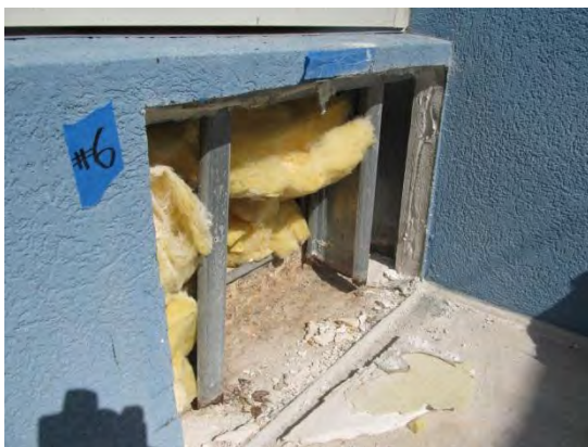
Photo #17 DTO #6 – Taken along west elevation.
