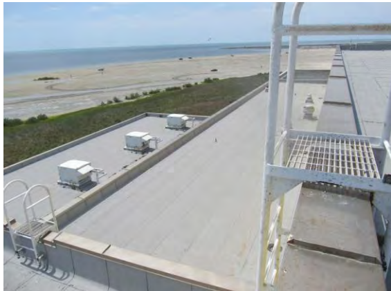
Photo #69 Overview of roof areas facing north.
