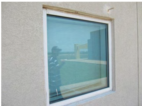
Photo #41 Typical "punch" window adjacent to Room 408.
