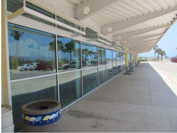
Photo #7 Storefront window system adjacent to lobby entrance.
