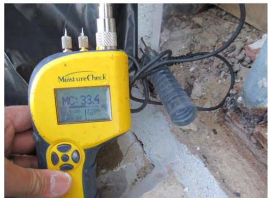
Photo #12 Qualitative reading (0-100 scale) of EPS insulation during spray testing.
