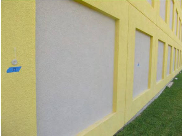
Photo #7 Overview of R7-R9 affixed to wall on east elevation.
