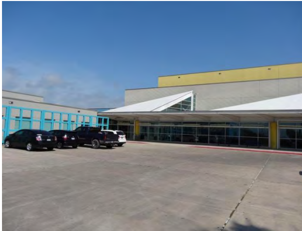
Photo #1 Overview of main entrance along the east elevation.
