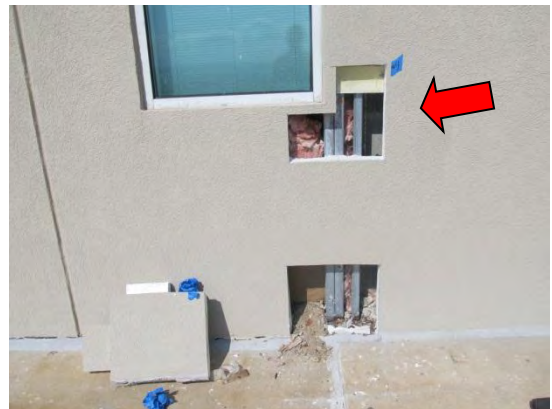
Photo #12 DTO #4 – Overview of #4 adjacent to window.
