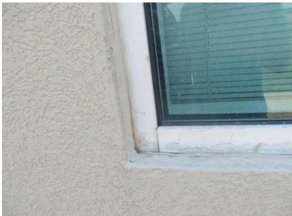
Photo #42 Sealant repairs and/or replacement along window perimeter.
