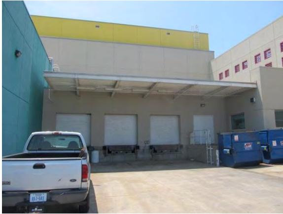
Photo #33 Receiving area along north side of facility.
