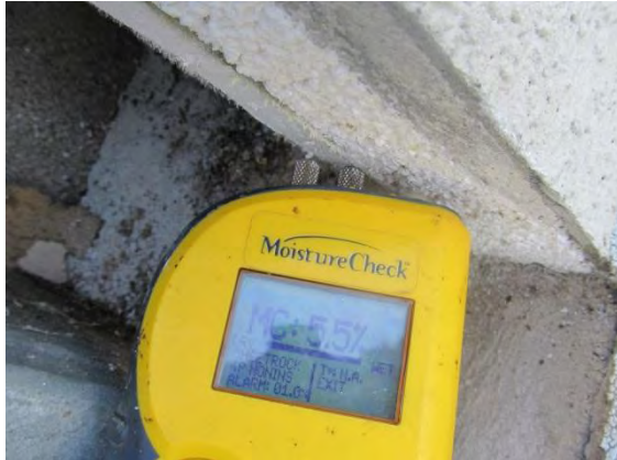
Photo #13 Moisture probe reading of exterior gypsum sheathing during spray testing.
