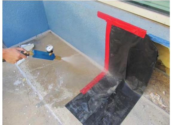
Photo #14 Water spray testing in progress at DTO #6.
