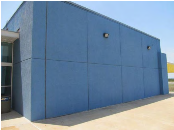
Photo #45 North elevation, Room 203.
