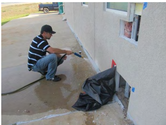
Photo #11 Water spray testing in progress on DTO #5.
