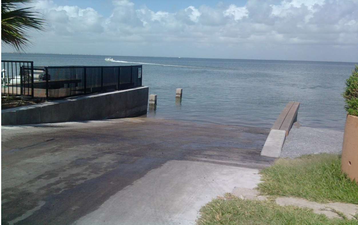
Recently completed Polaris Street Boat Ramp
