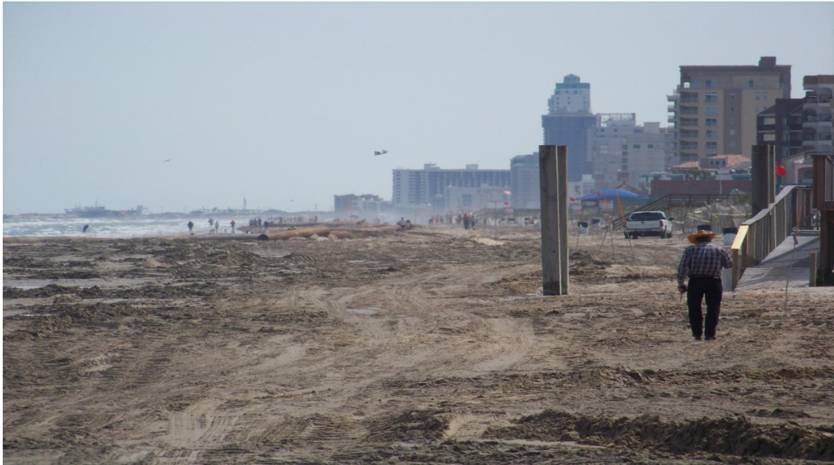
Re-nourishment from dredge material
