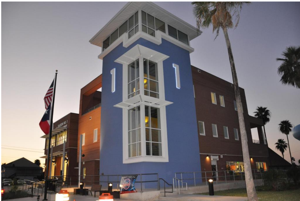
Completed Fire Station
