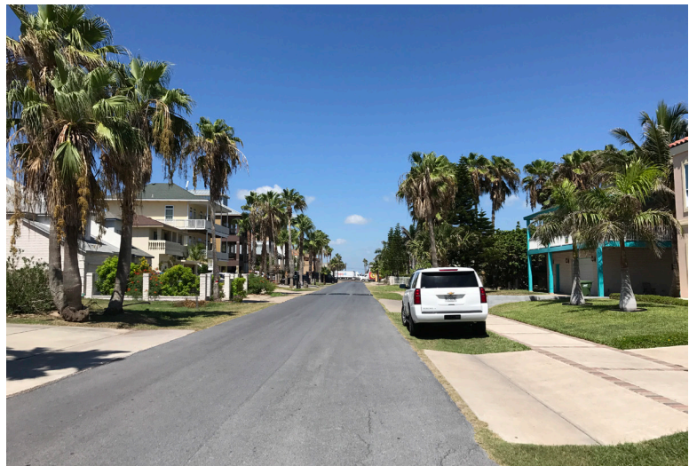
Existing Sidewalk on E Red Snapper St
