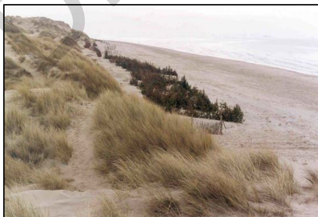
Figure 16: Typical Christmas Tree Placement (Pye et al, 2007)
