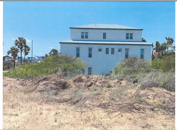
View of left adjacent lot
