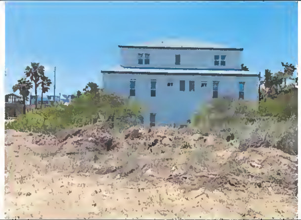
View of left adjacent lot
