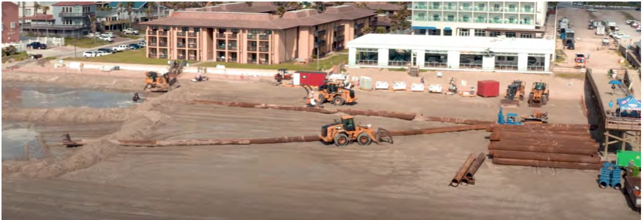
The Shoreline Department in partnership with the U.S. Army Corps. of Engineers, GLO, and Cameron County work to renourish the beach.
