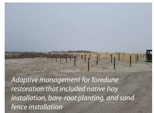
Restored foredune 6 months after project completion
