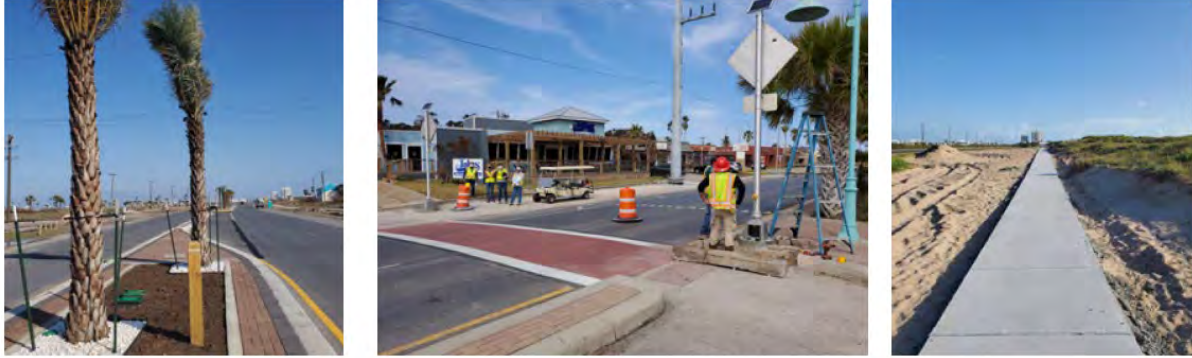
The PR 100 Median, Boardwalk, Sidewalk, and Traffic Signal Improvement Project
